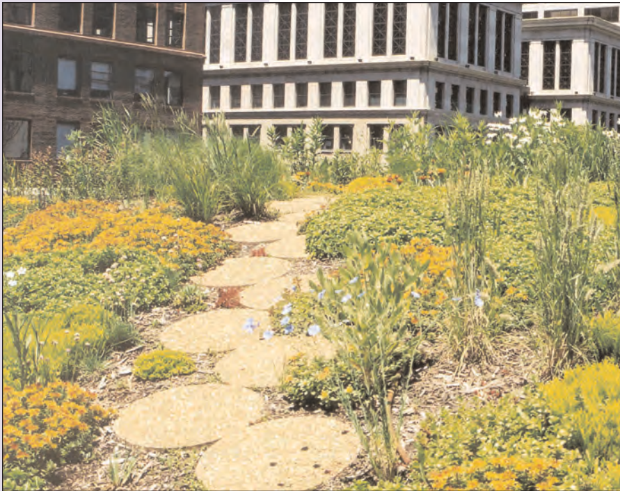
Green roof close-up, showing variety of plant material and stepping stones for access to the garden.
